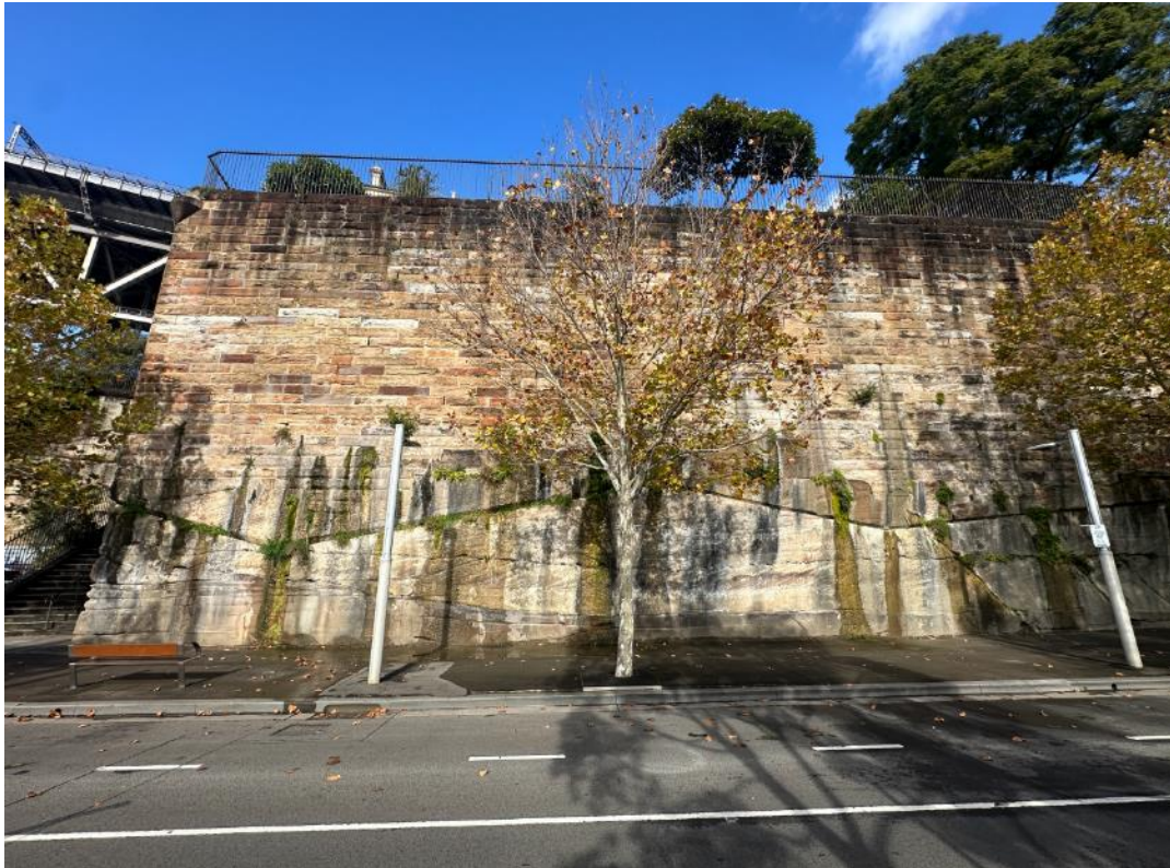
Figure 11: Western boundary of 'Milton Terrace' to the south of the site viewed from Hickson Road
